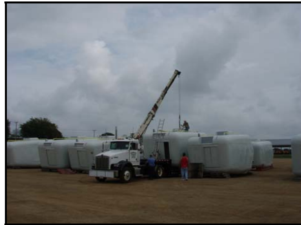
Fully assembled nacelles awaiting transport
