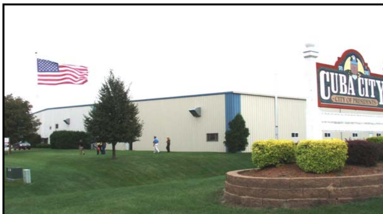
Wausaukee Composites' dedicated wind turbine component plant in Cuba City, Wisconsin
